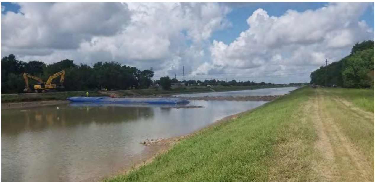
Figure 2 - Current Work Area (Station 140+00) - Staging Cofferdams Looking Back towards Canyon Gate
