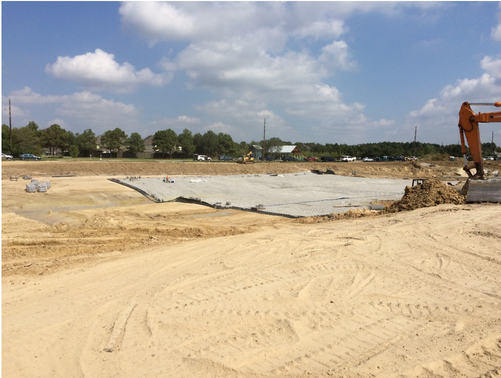
Figure 13 – Looking at ACBs from Top Bank Looking Toward Exploration Park, Northeast (Construction)
