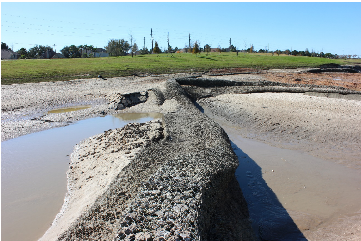
Figure 10 – East of the Sanitary Sewer looking Southwest at the Bottom Alignment of Gabions
